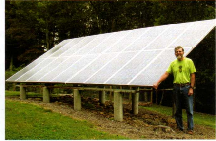
Dr. William Baker's 18-solar-panel array for his home in Montgomery County has produced about 18,000 kilowatt hours since 2004.
