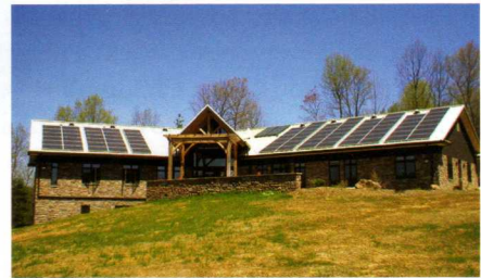
The administrative offices of Wall Residences in Floyd, VA, have a 15-kilowatt system consisting of 82 solar panels, the largest photovoltaic array in the region.
